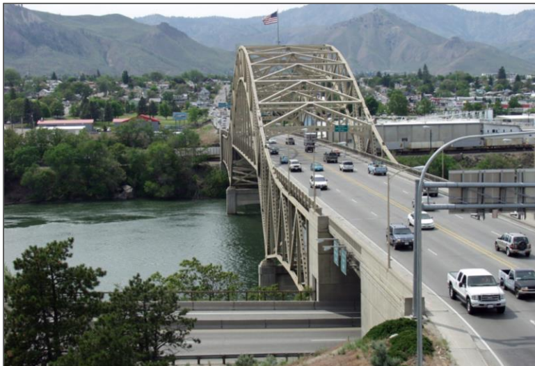
Figure 10 – Typical Street Truss Style Bridge Constructed in 1950 (WSDOT)
