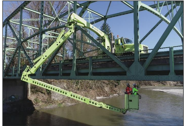
Figure 20 – Under Bridge Inspection Truck (UBIT)
