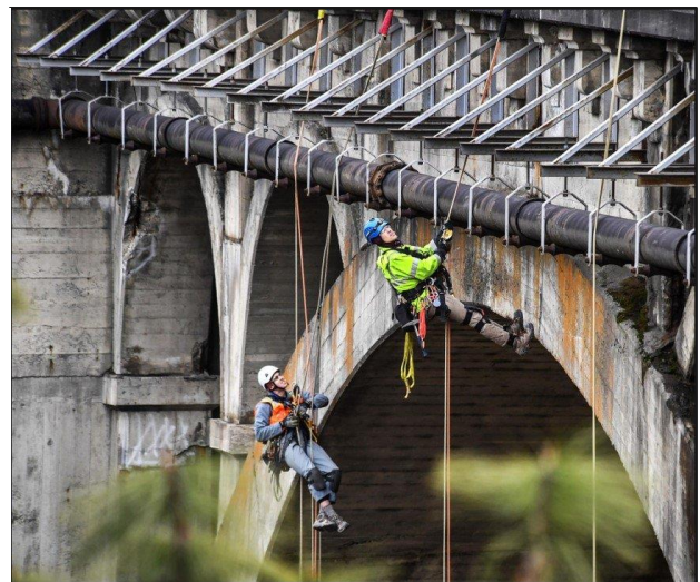
Figure 21 – Rope Access Inspection Team
