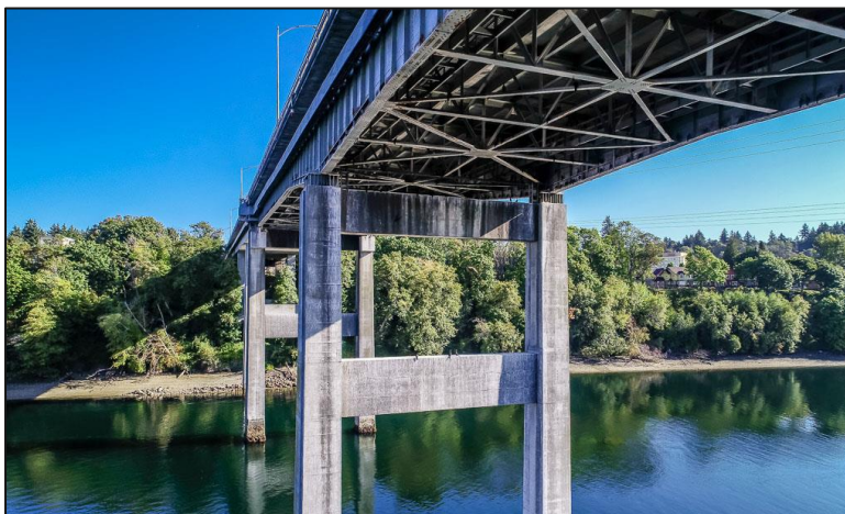
Figure 11 – Steel Plate Girder on the Warren Avenue Bridge
