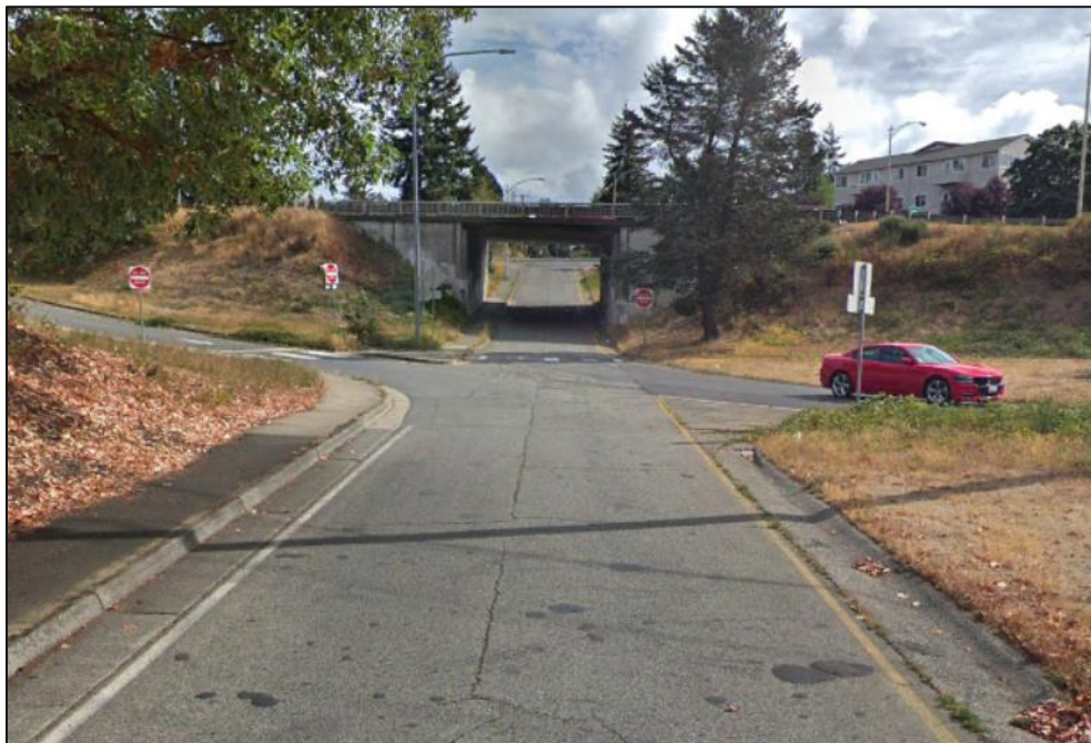
Figure 7 – Callahan Drive (Looking East toward Warren Avenue)
