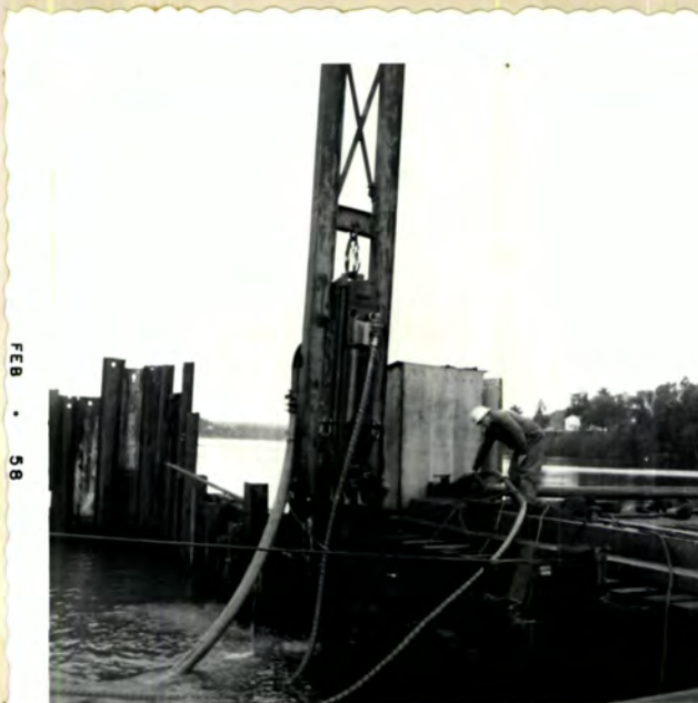
DATE: FEBRUARY 19, 1958 REMARKS: Pile driver at Pier No. 5 cofferdam.
