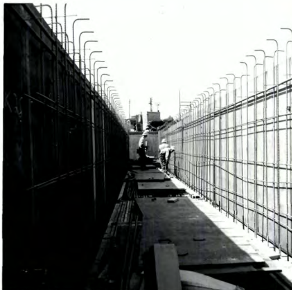
DATE: JULY 10, 1958 REMARKS: Removing falsework bents from span no. 8 with water rig.
