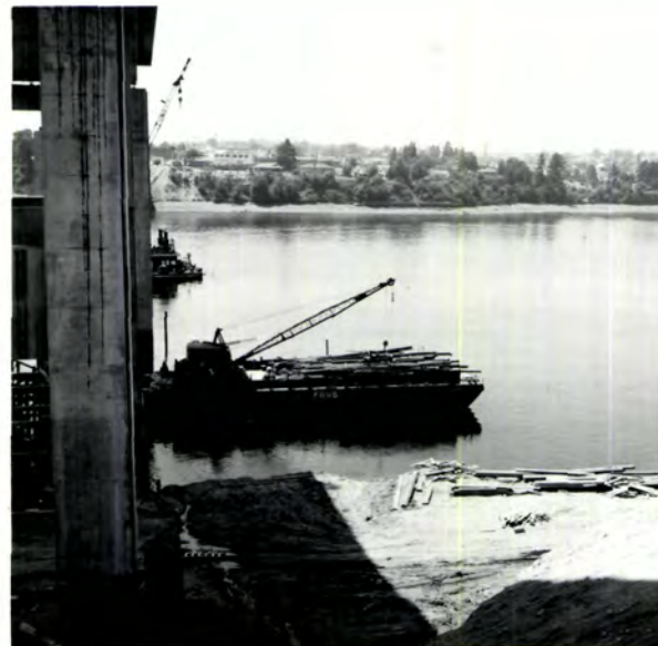
.....DATE: JULY 10, 1958 REMARKS: Setting one of the last falsework bents on span no. 4. with water rig.
