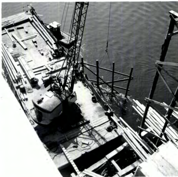
.....DATE: JULY 10, 1958 REMARKS: Setting one of the last falsework bents on span no. 4. with water rig.
