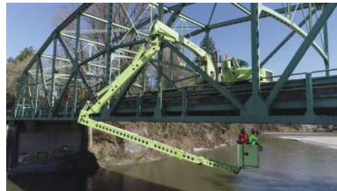
Under Bridge Inspection Truck (UBIT) Deployment
