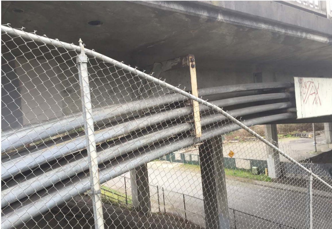
Figure 7: Electrical Conduits
