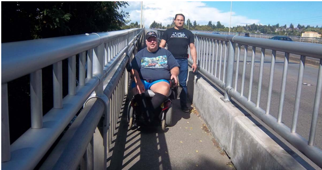
Figure 1: Photo of Narrow Walkway
