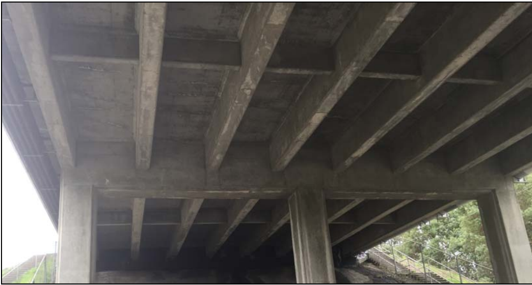
Figure 11: Concrete Tee-Beam Photo
