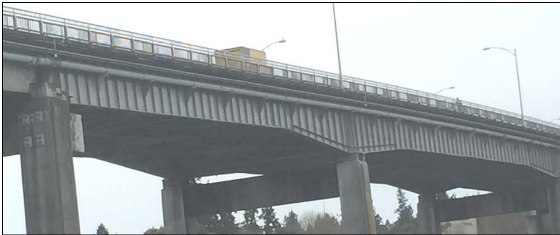
Figure 15: Steel Plate Girder Photo
