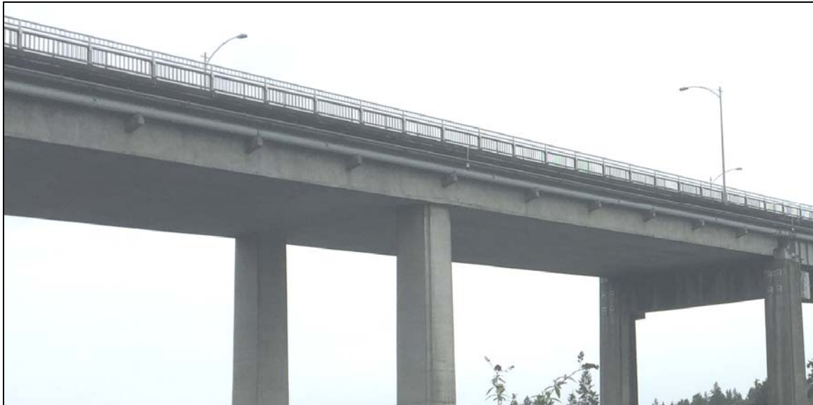
Figure 13: Concrete Box Photo
